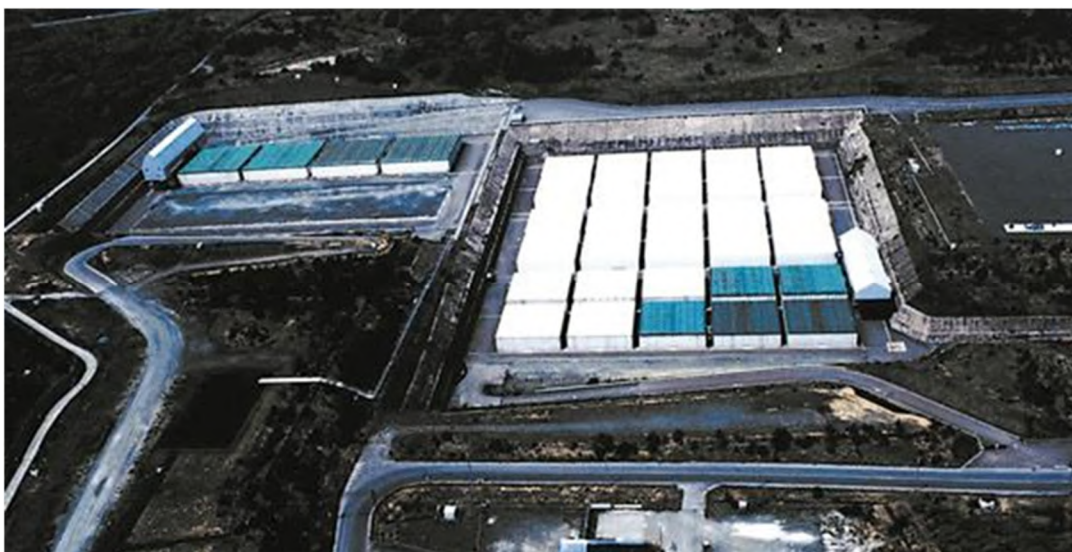
Fig. A12-2 Japan Nuclear Fuel Ltd. Low-level Radioactive Waste Disposal Center
